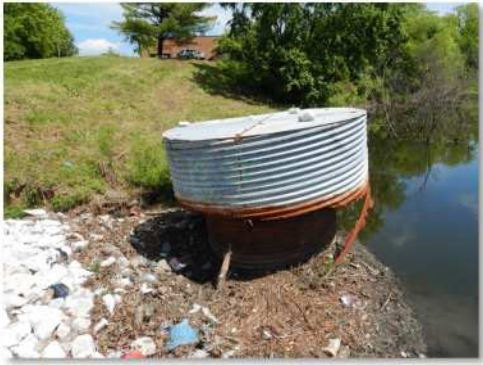
Pic. 1. Deteriorated barrel of the principal spillway being covered by riprap.
