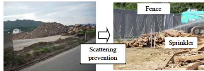
Photo 4 Fence and sprinkler at tentative storage to prevent scattering of airborne
