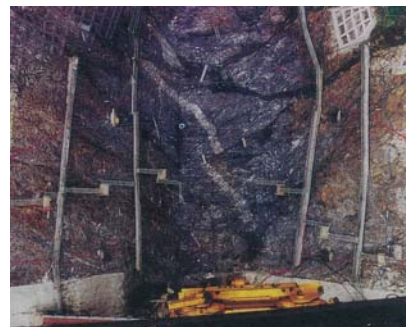
Figure shows that an excavated base for the Mikawasawa Dam exposes Mesozoic sandstone and shale with porphyrite intrusion, which belong to the Ashio Accretionary Complex located in the northern Kanto district in Japan.
