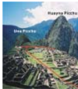
Machu Picchu Landslide (Sasa et al., 2002)
