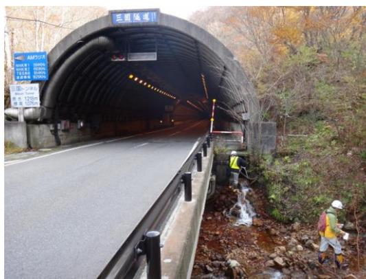
Photo. 1 Acid drainage water from a tunnel
