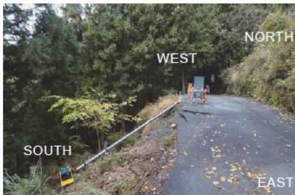
Photo1 Deformation appeared on the surface of the road in Landslide block II area.
