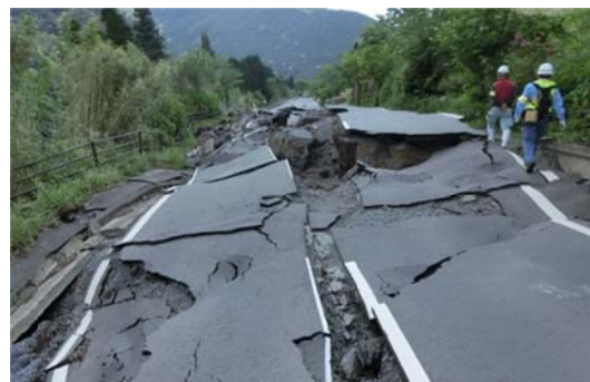
Investigation of the Earthquake
