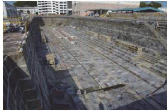
Fig. 1 Yokosuka Arsenal No.1 Dry Dock
