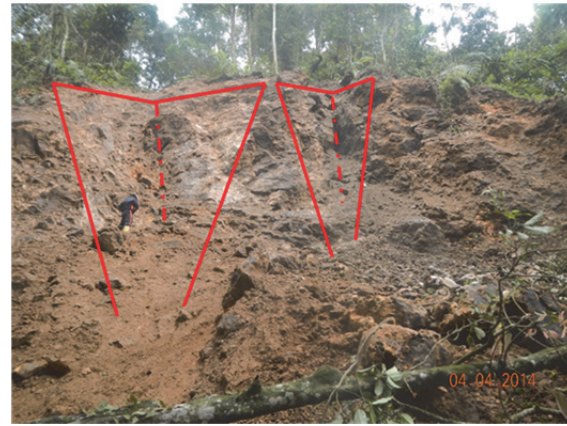
Fig. 2 Wedge failure on the Southern Slope
