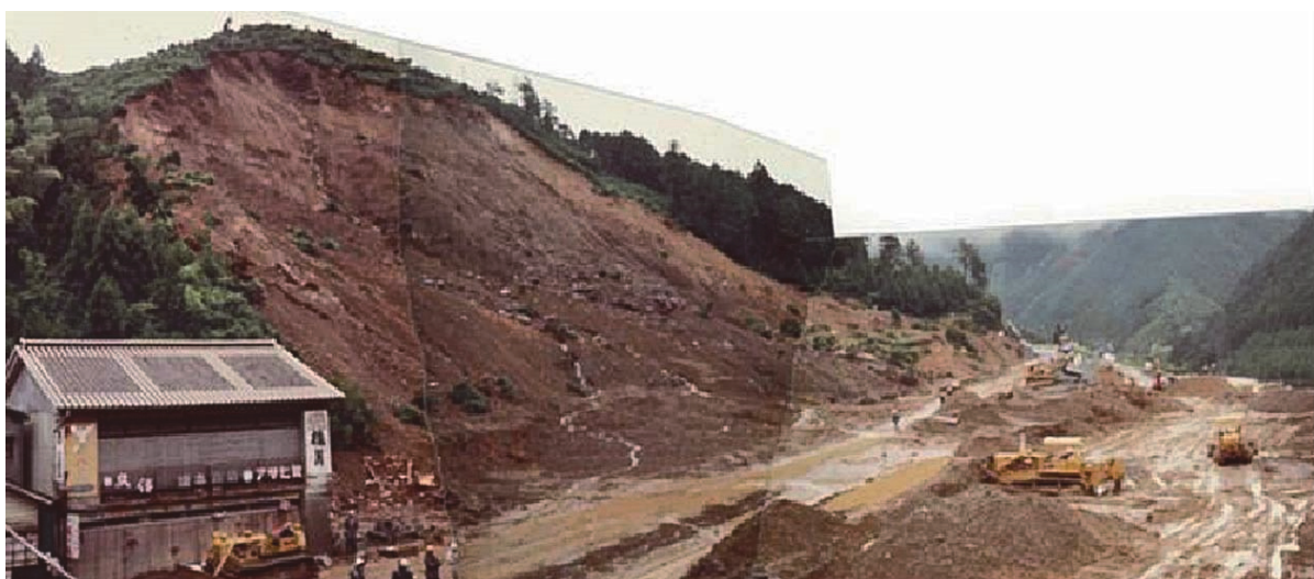
Photo.4 : Shigeto Station six days after the disaster on July 11, 1972. The station facilities and the stopped train were washed away by slope collapse (Photograph by OYO Corporation)
