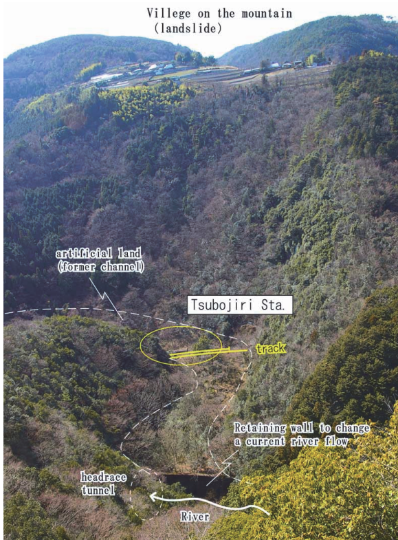
Photo.2 Overlooking view of the Tsubojiri station and the landslide on the mountain (Kato, 2013)
