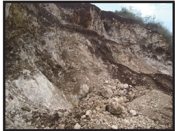
Photo 1. Local failure at Site X03 with 53° slope angle
