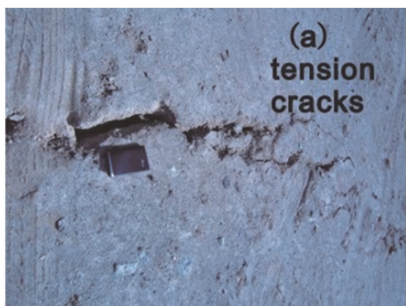
Fig. 3 Tension cracks
