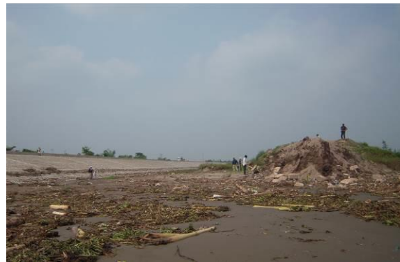
Fig. 3 Broken seadyke in Hai Hau
