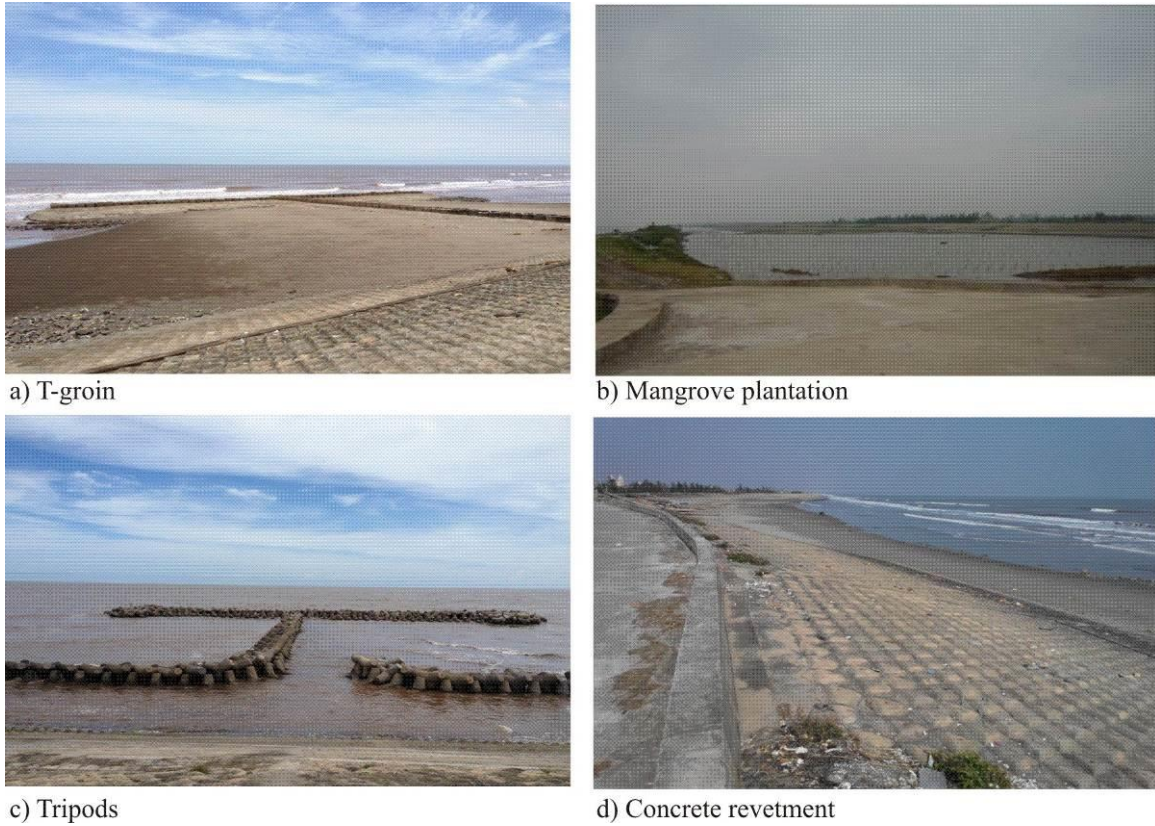
Fig. 4 Conventional measures in Hai Hau coast
