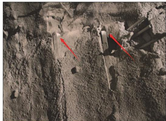
Photo.3 Failure rock mass and steel arches in side wall at DIK76+558
