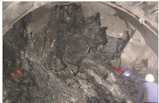
Photo.4 1# (left) and 2# (right) borehole camera observation holes at DIK76+543
