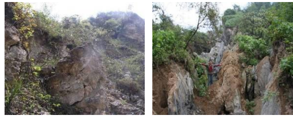
Fig. 13 Collapse induced by the slope rockmass were shattered
