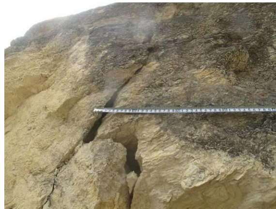
Fig. 4 Seismic fracture throughout inside rockmass
