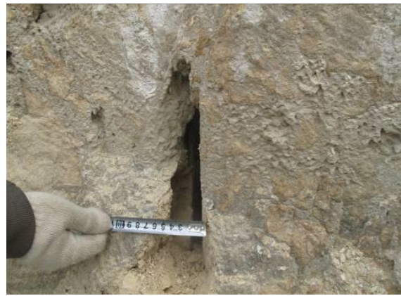
Fig. 8 Closure type seismic fracture
