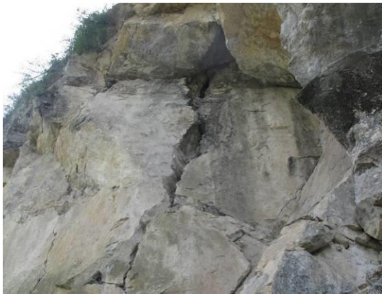
Fig. 9 Extended type seismic fracture
