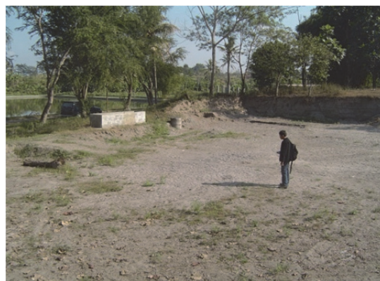
Figure 1. Liquefaction evidence due to Yogyakarta Earthquake
