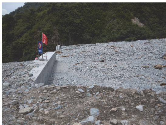
Fig.9 The No.5 dam was filled up again after the reinforcement and restoration in 2004(2014-7-14)
