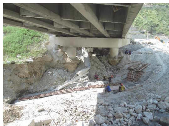
Fig.5 Bare pier washed by debris flow under a bridge on Dujiangyan-Wenchuan freeway
