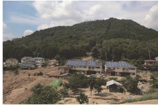
Photo 4. The distant view of landslide
