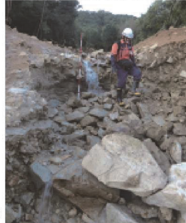
Photo 5. Erosion and sediment area of landslide
