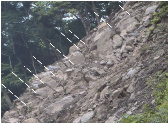
Photo 2 Open joints in the rock slope at the failure shown in Photo 1 (white broken lines)
