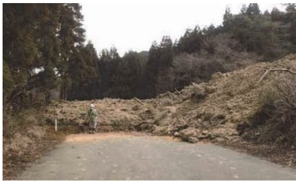
Photo 18 A case of failure of embankment which filled a road
