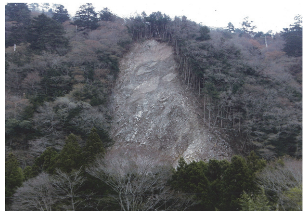
Photo 3 A case of rock slope failure in the Mesozoic granodiorite area
