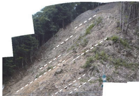
Photo 4 Joints of dip slope in the rock slope at the failure shown in Photo 3 (white broken lines)
