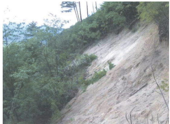
Photo 10 Upper part of the failed slope shown in Photo 9
