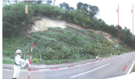
Photo 9 A case of soil slope failure on a cut slope in the Mesozoic granite area
