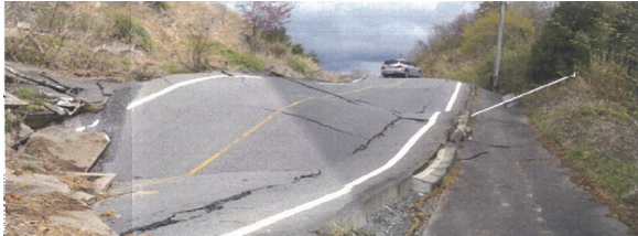
Photo 13 Uplifted road at the toe of the landslide shown in Photo 11
