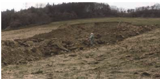
Photo 19 Upper part of embankment failure shown in Photo 18
