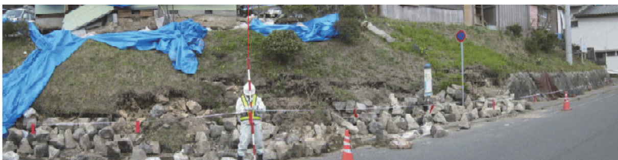
Photo 21 A case of failure of masonry wall near the road
