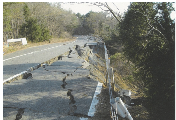
Photo 16 A case of failure of embankment constructed filling a valley
