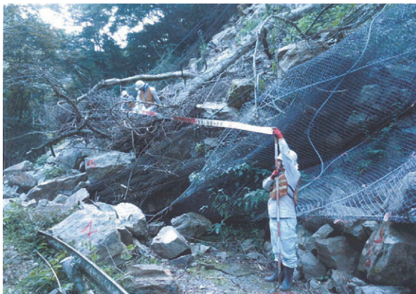
Photo 1 A case of rock slope failure in the Mesozoic schist area
