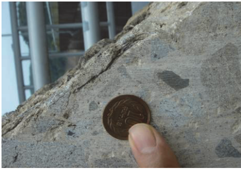
Photo.7 Crack and pop up of dam concrete. (The aggregate contains laumontite.)
