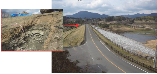
Photo.6 A rock fill dam after repaired laumontite bearing rip lap rock. (Left photo is trench investigation for checking deterioration.)
