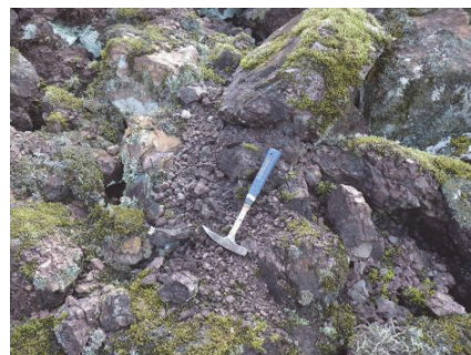
Photo.5 Deterioration of rip lap of rock fill dam by freezing and thawing
