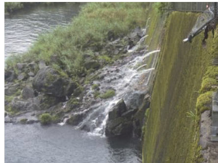
Photo.3 Leakage water from dam
