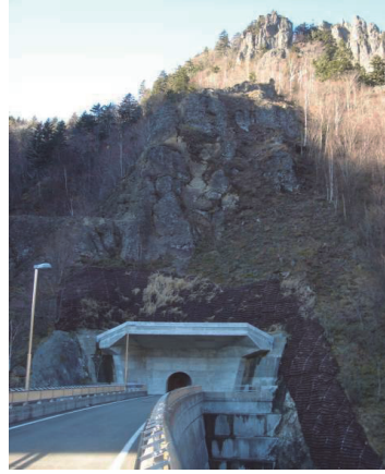
Photo.9 Rock shed on a dam crest
