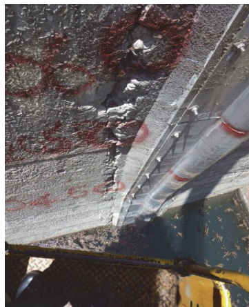
Photo.1 Open crack along a transvers joint
