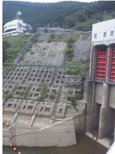
Photo.10 Landslide near a dam
