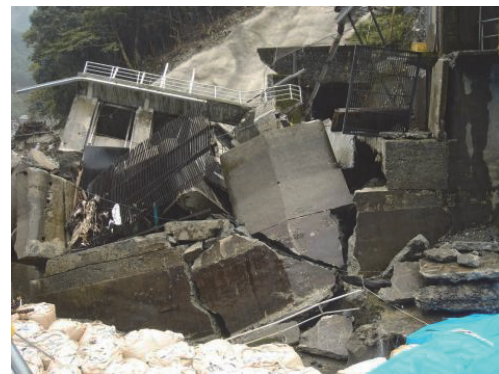
Photo.4 Collapse of a weir by erosion of foundation
