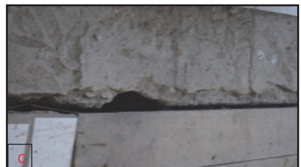
Figure 5. A,B,C. Impact of Creep Movement
