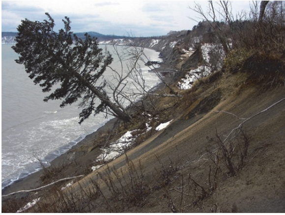
Fig. 2 Ongoing landslides in hillsides of Akkeshi Bay.
