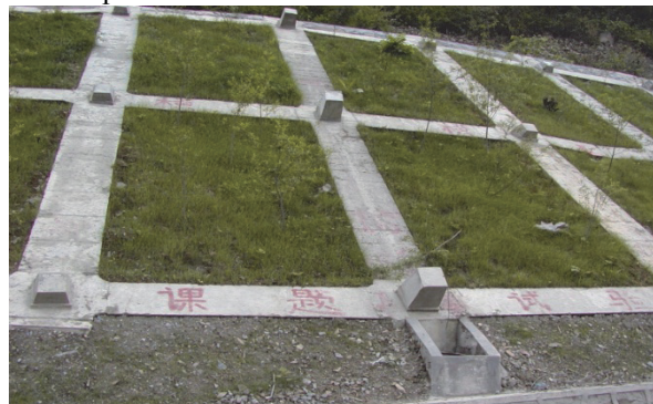
Fig.5 Prestressed anchor cable frames
