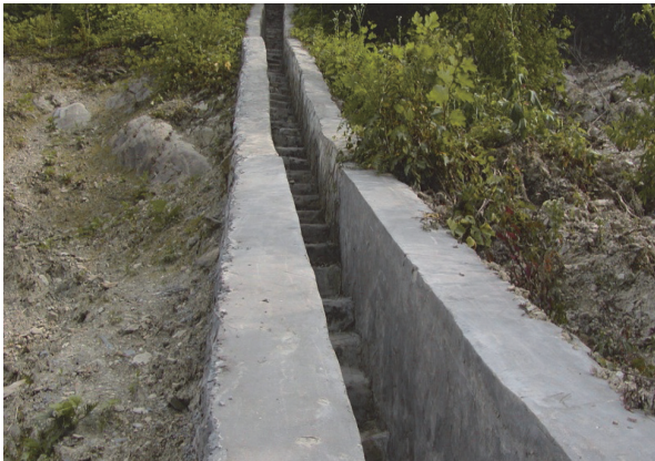
Fig.7 The rapid stream slot for drainage
