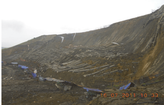
Fig. 5 The failure condition of the anchor cable frames
