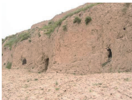
Fig.3 Sinkholes in the leading edge and backscarp of Shijiaping Landslide
