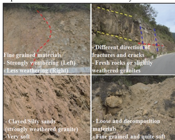
Fig. 6 Materials of weathered granite rocks slide. In addition, in the layer of high permeable
