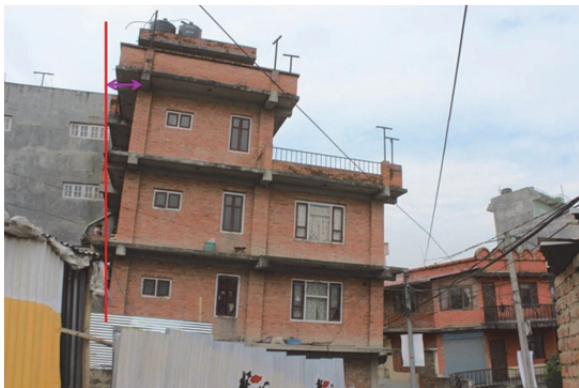
Photo. 8 Land subsidence and tilting of house due to liquefaction of lower strata
