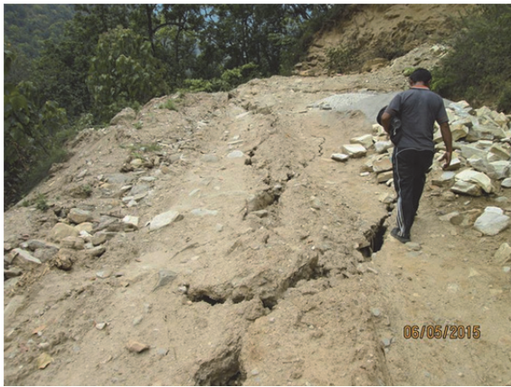
Photo. 7 Failure in Cut-and-fill part of rural road
