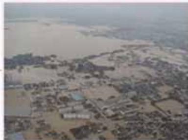
Flood (White Paper on Land, Infrastructure and Transport in Japan, 2005)
